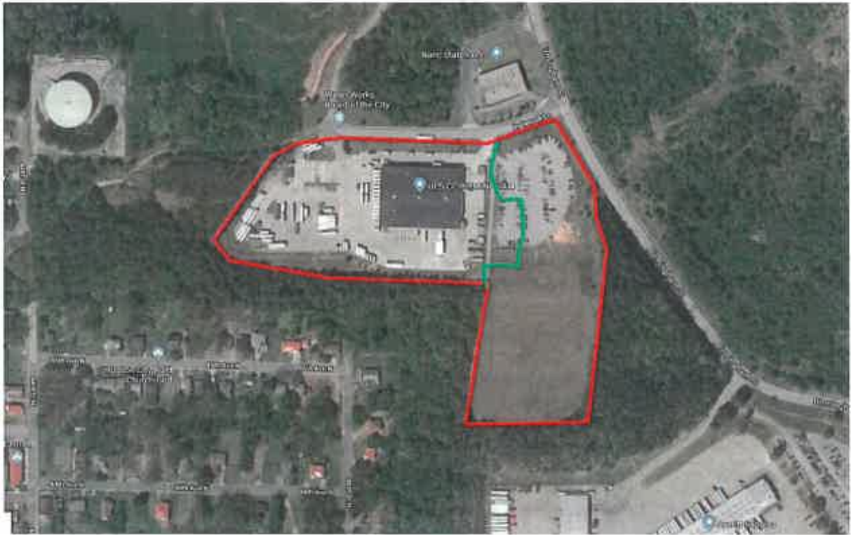
Existing Fencing Present
