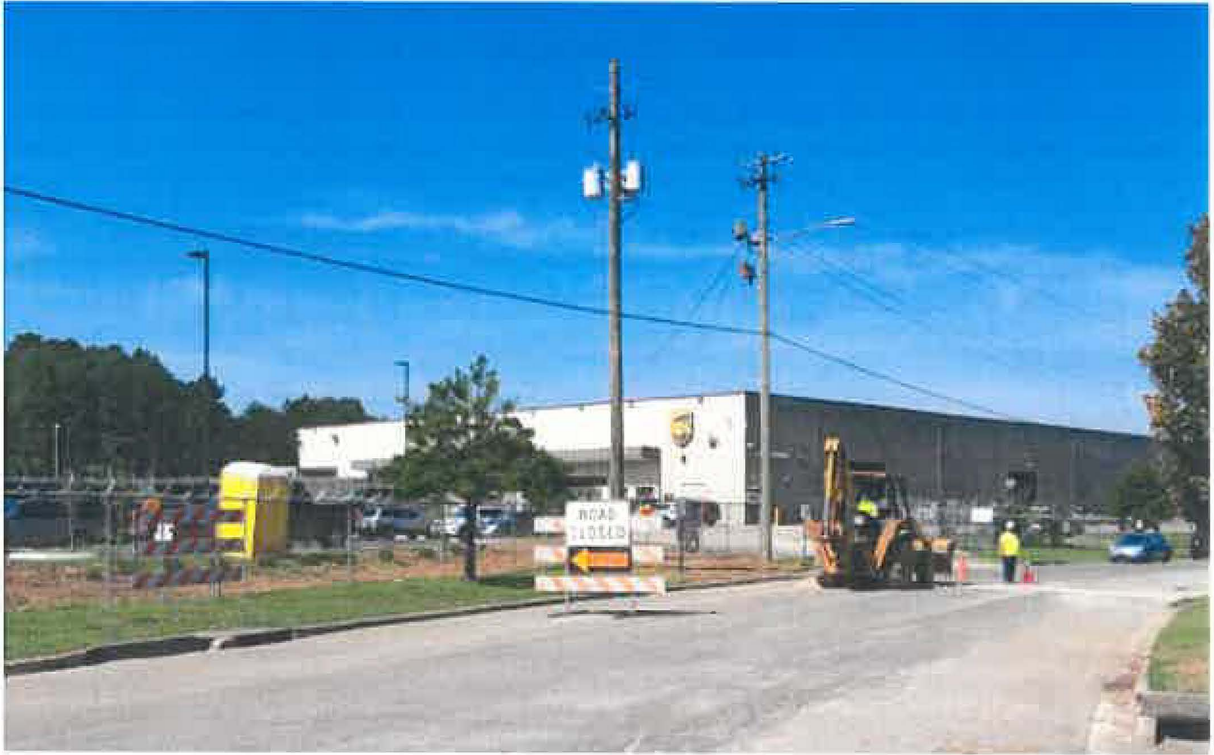
Existing Fence at Front of Property
