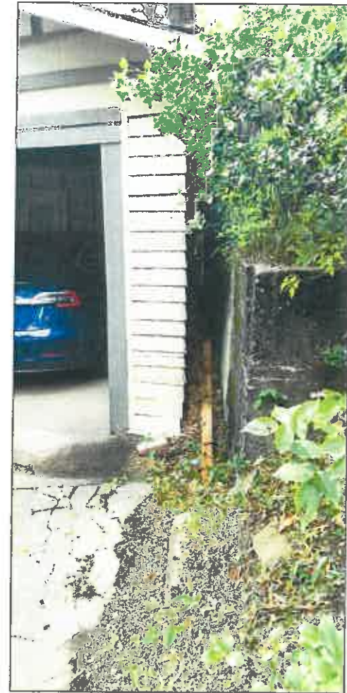
CLOSE-UP VIEW OF EXISTING GARAGES PROXIMITY TO EXISTING RETAINING WALL
