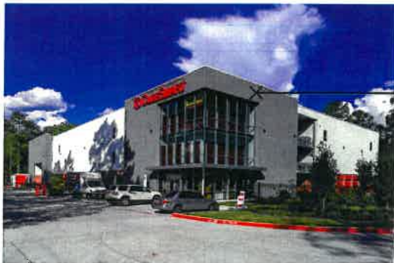
SECOND SET OF PROPOSED CHANNEL LETTERS WILL MOUNTED TO THIS FASCIA
