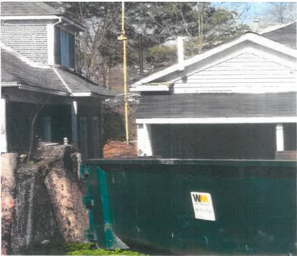
East side yard view
