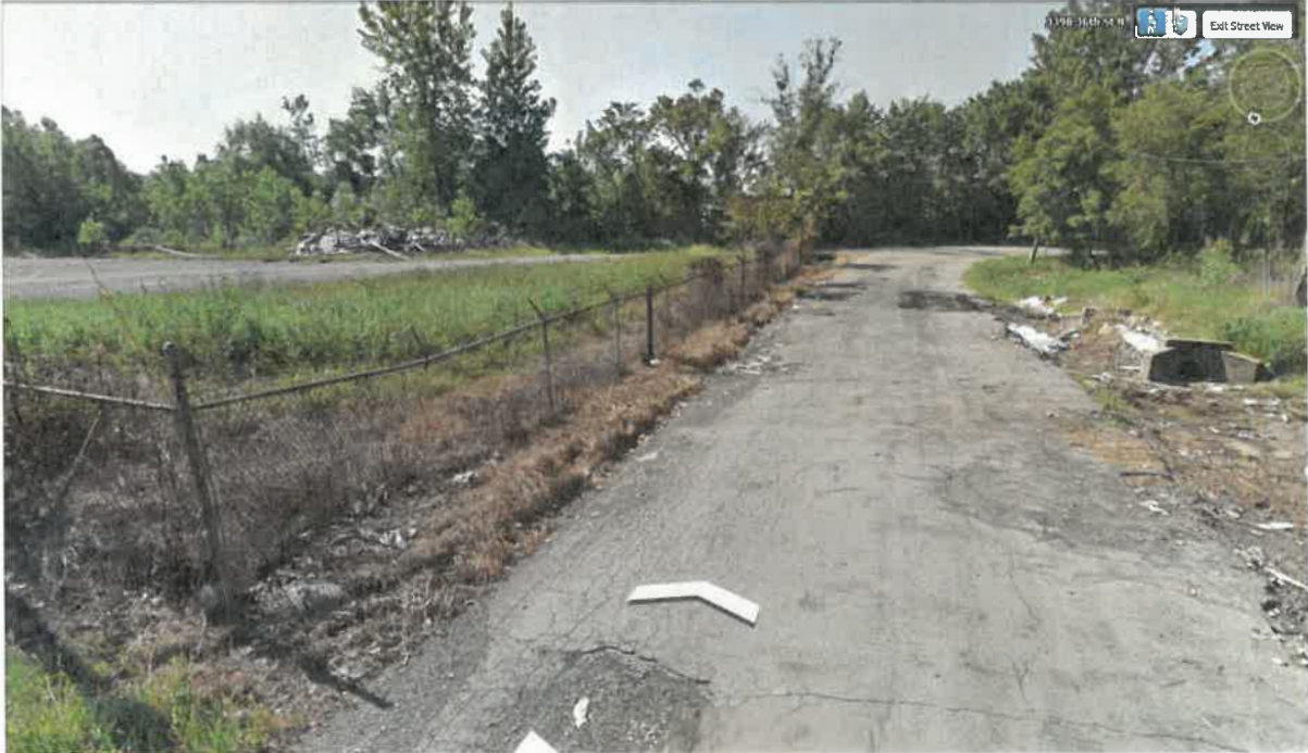
Fencing along 36 th St
