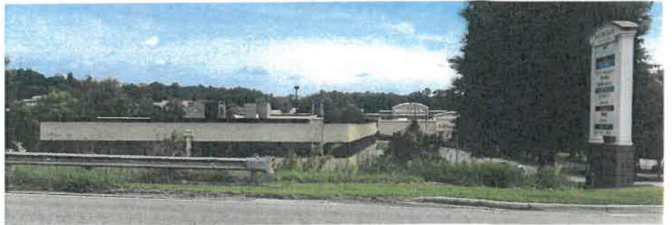
Building Side Also Visible from 280
