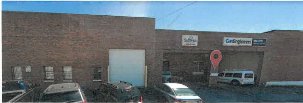
2ND AVE. S. (SULLIVAN BUILDING TO BE DEMOLISHED FOR COURTYARD)
