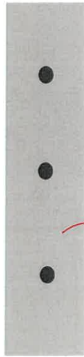
Wall with holes drilled into it to receive signage
