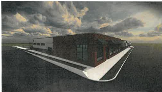
CORNER OF 17TH STREET S. AND 2ND AVE. S.
